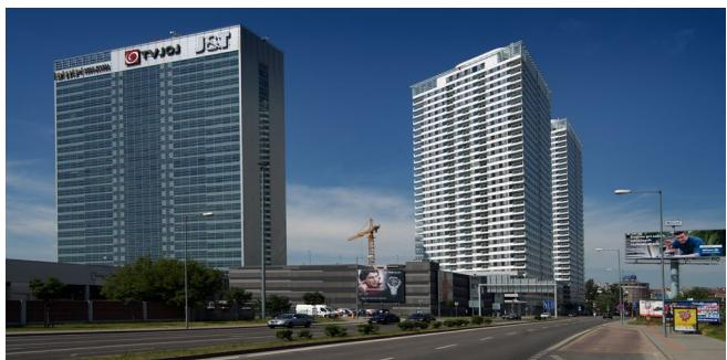
Within the first stage of Panorama City, Chemkostav carried out a rough construction consisting of earthworks, piloting, reinforced concrete structure and superstructure made of steel construction. A total of 6.500 tons of iron and 45.000 m<sup>3</sup> of concrete were used on the site, the towers are based on nearly 500 piles reaching the depth of up to 24 meters.
